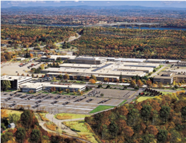
Aerial view- TechCity is located between New York City and Albany, NY.
